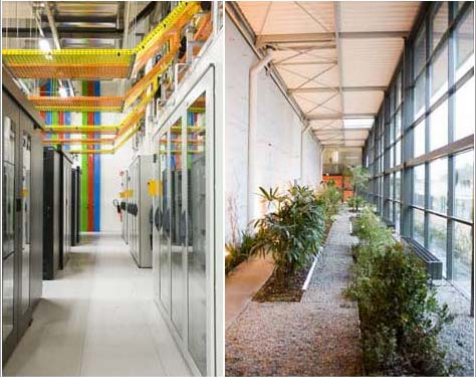
Waste heat from servers at the new Telety Paris data center (left) is being used to heat an on-site arboretum (right).
